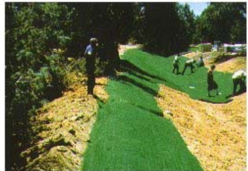
June, 1995 Installation of Landlok TRM 450
