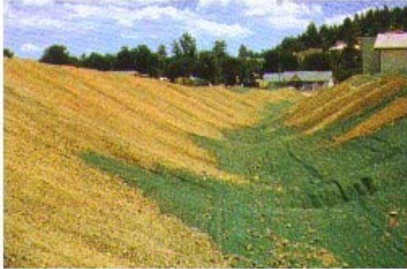
The TRM was soil-filled to maximize performance.
