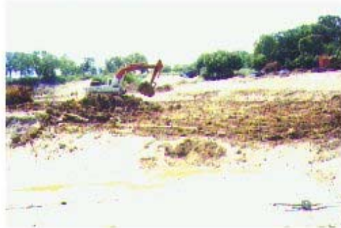
Workers excavate Sims Bayou in preparation for the project
