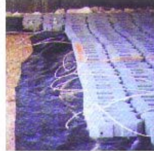
Close-up of cellular concrete mat system with Geotex 104F geotextile underlayment.
